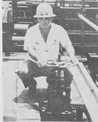
GEORGE A. Larmonie is standing by the tie-in which he suggested be installed to maintain ship fuel loading rates.
